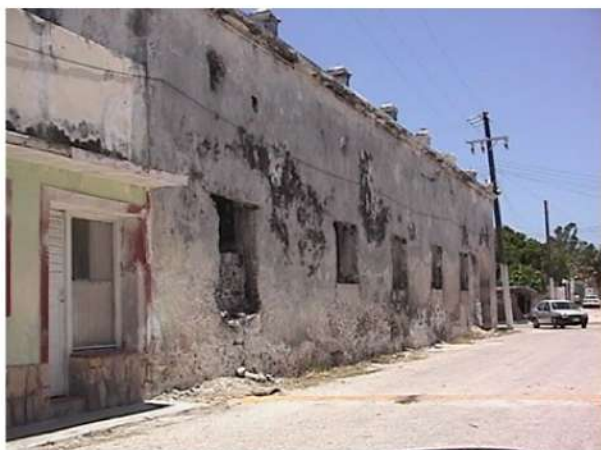
The old Customs Office in Sisal now abandoned.
